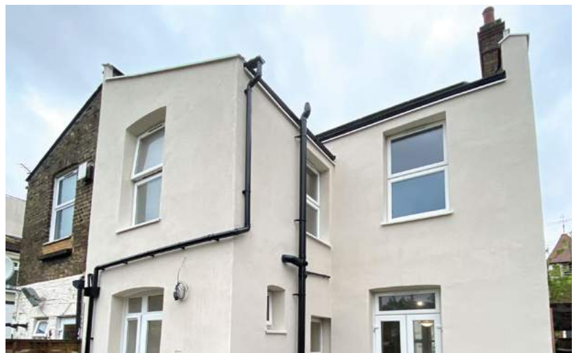
Final render on the external wall insulation
