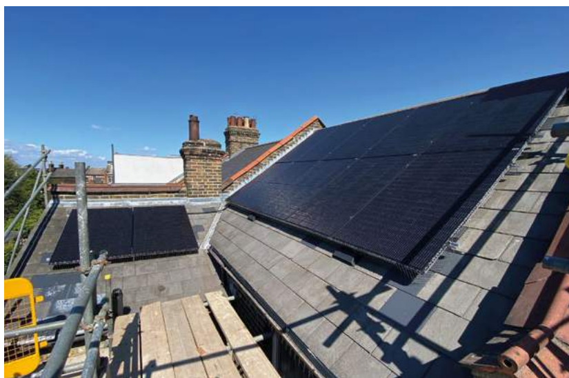
Installation of 12 photovoltaic solar panels
