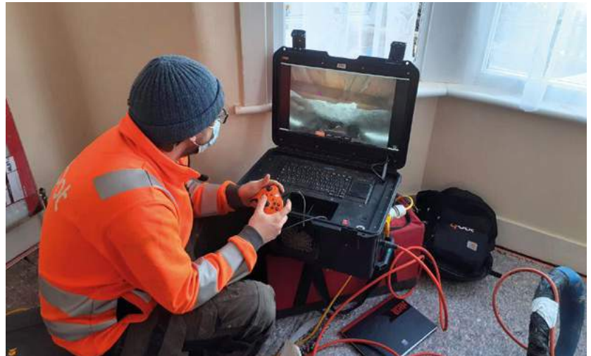
Robot being controlled to spray insulation foam under suspended floor
