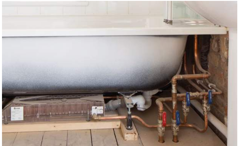
Zypho bath tub system being installed
