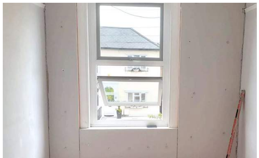
Installation of the internal wall insulation
