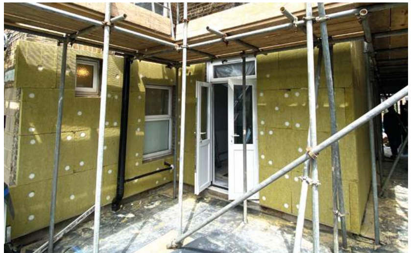
External wall insulation being installed
