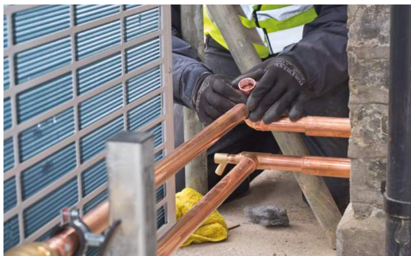
Installing a Vaillant aroTherm heat pump
