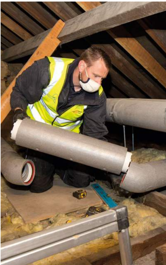
Installation of ductwork
