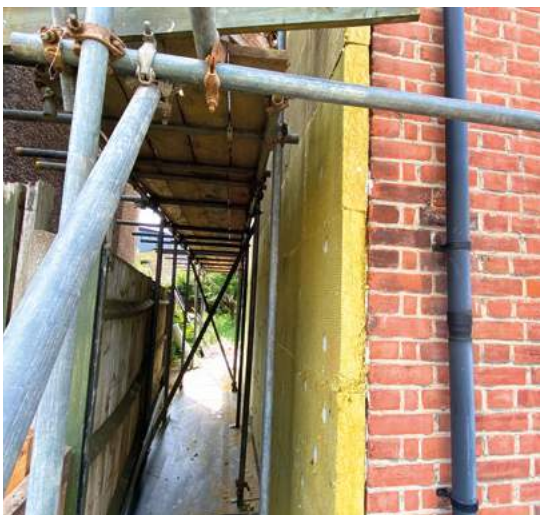
External wall installation against the existing house
