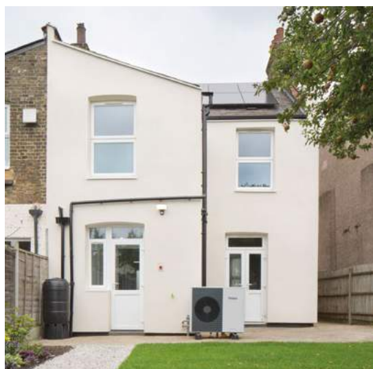
Heat pump in position
