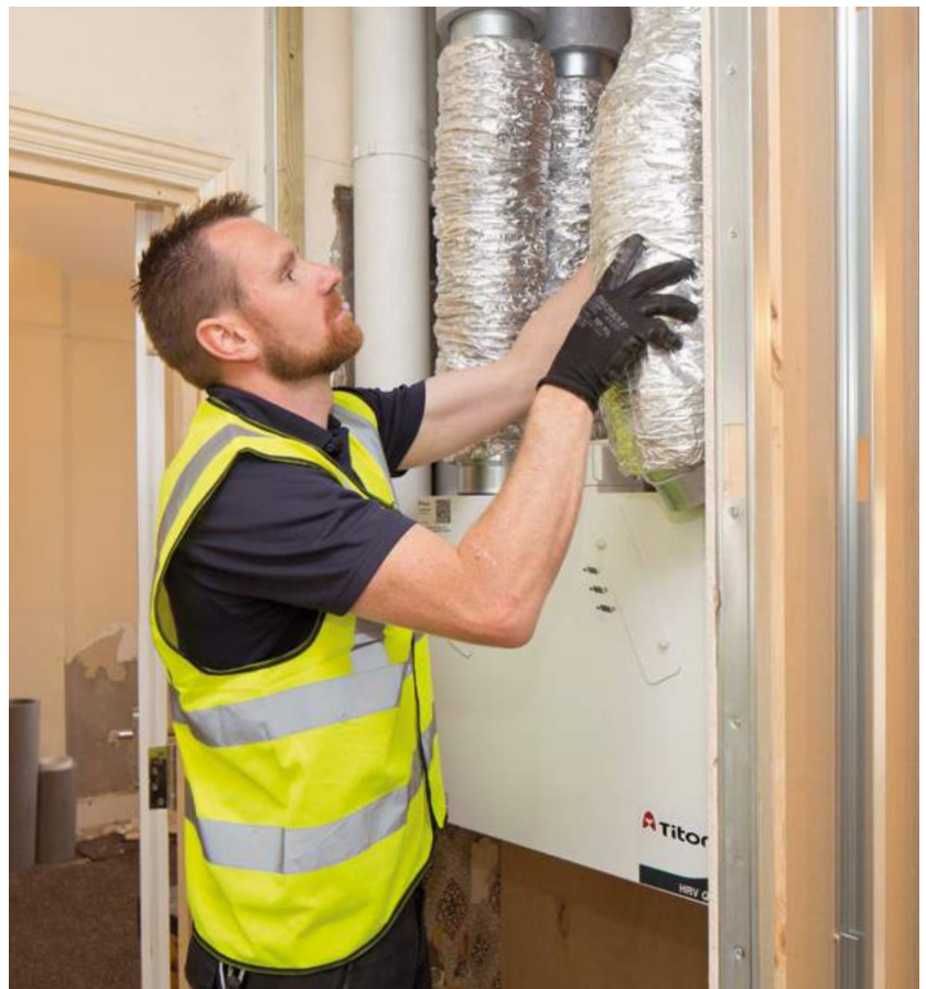
Installing a Titor 1.6 mechanical ventilation heat recovery unit
